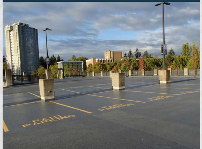
Left: Old concrete slabs and insulation removed before deck repairs and membrane replacement
