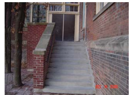
Stair after replacement
