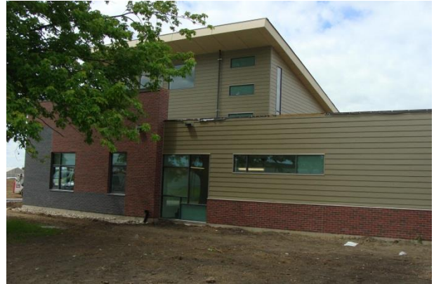
Side elevation of the building addition
