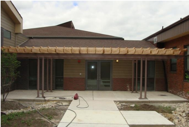
Exterior courtyard and pergola canopy between the original building and the new addition.
