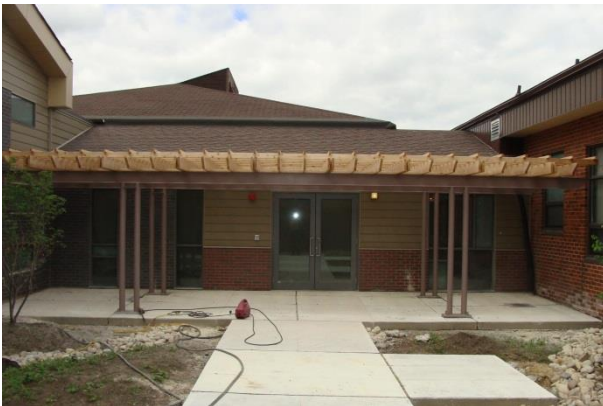
Exterior courtyard and pergola canopy between the original building and the new addition.
