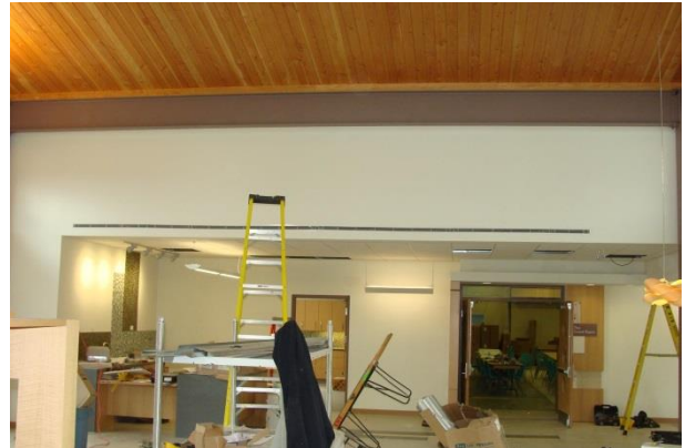
New main lobby interior including wood deck ceiling.
