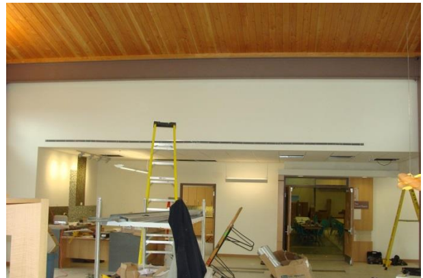
New main lobby interior including wood deck ceiling.
