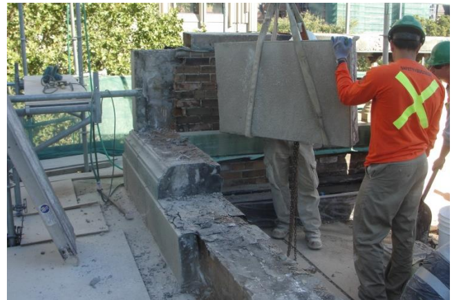
Stone Parapet Restoration in Progress
