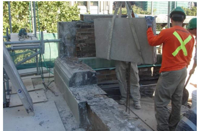
Stone Parapet Restoration in Progress
