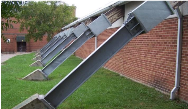
Final condition of remediated beam
