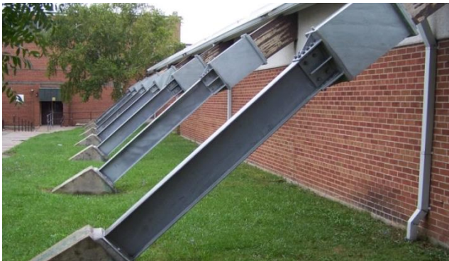
Final condition of remediated beam
