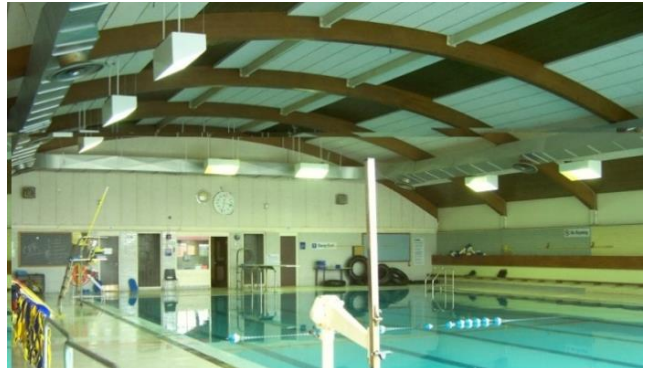
Final interior condition
