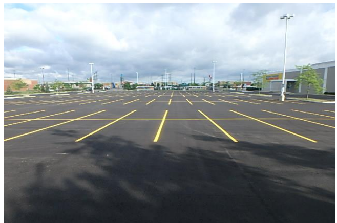
New Asphalt Pavement
