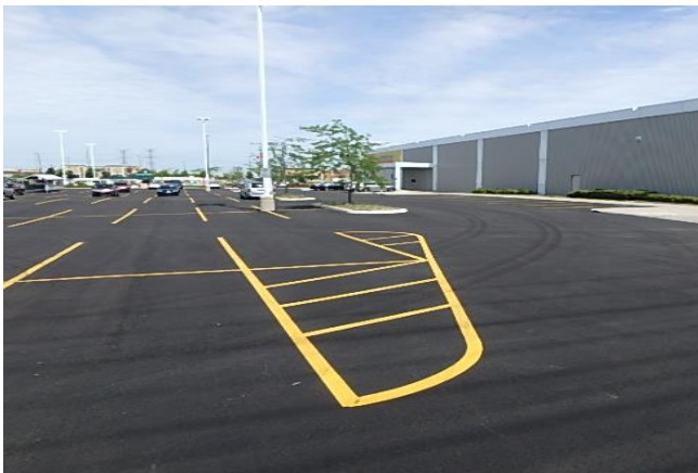
Concrete Island Removed to Accommodate Trucks Turning Radius
