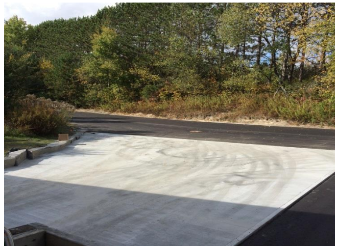
New Concrete Pad and Asphalt Pavement
