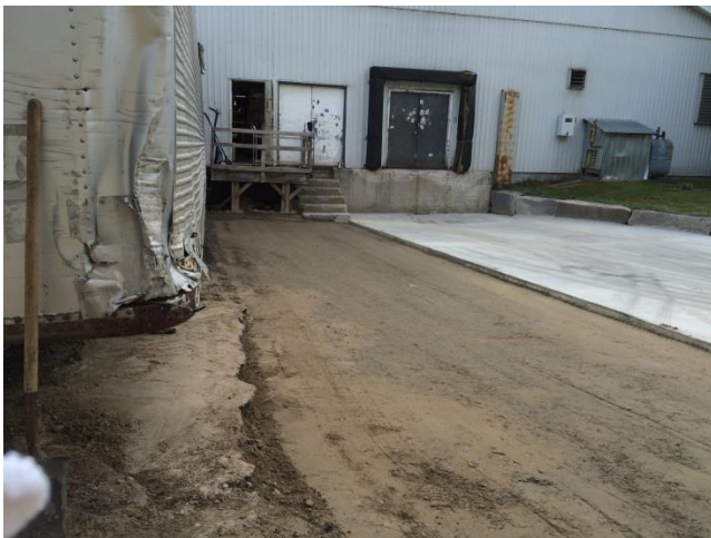
New Concrete Pad and Asphalt Pavement
