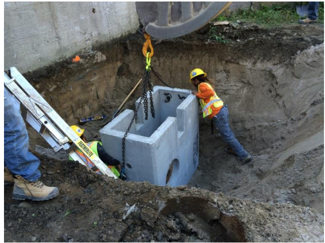
Installation of Double Catch Basins at Loading Dock
