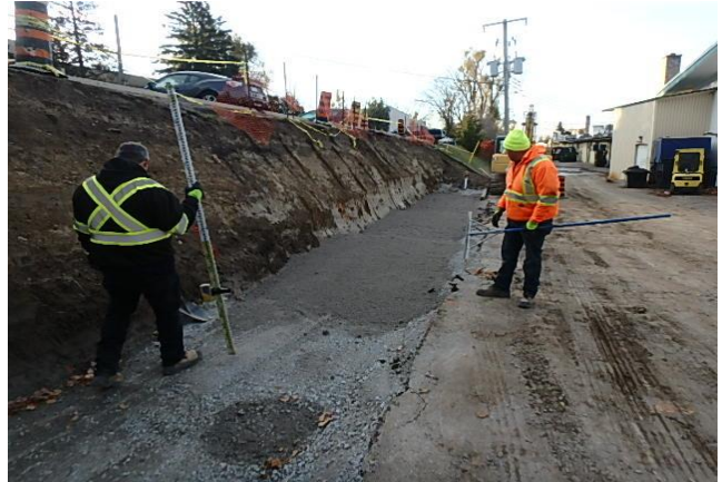
Preparation of Base and Subbase for the Retaining Wall
