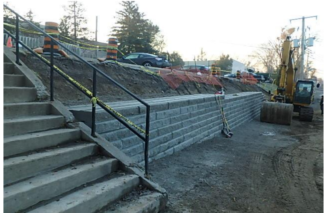
Widening of the Loading Area to Accommodate Trucks Turning Radius
