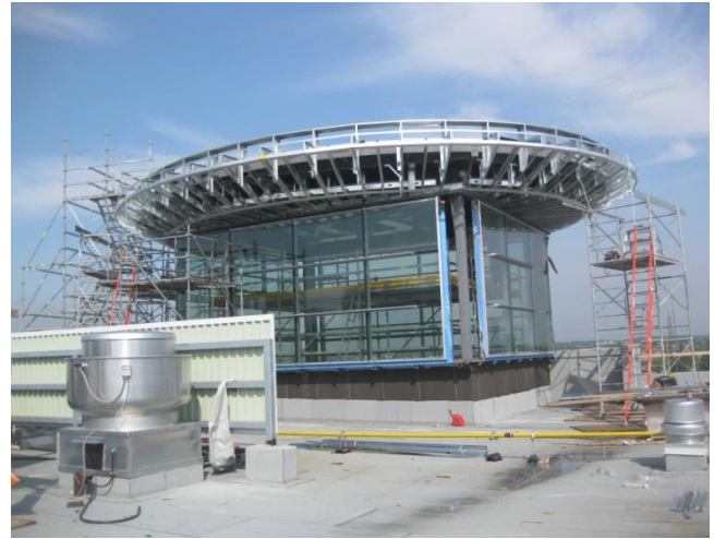
Construction of new entrance feature
