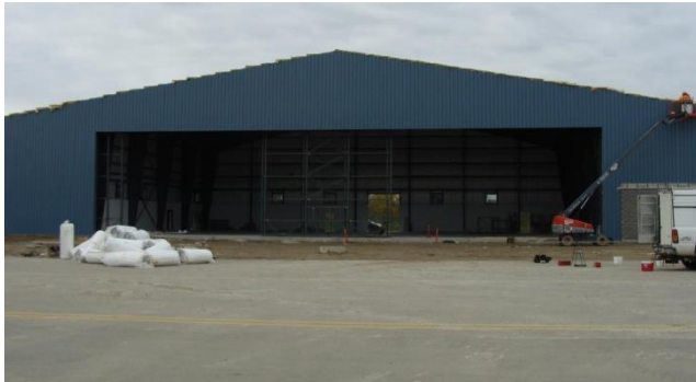
Endwall elevation (airside) with exterior cladding installation being completed
