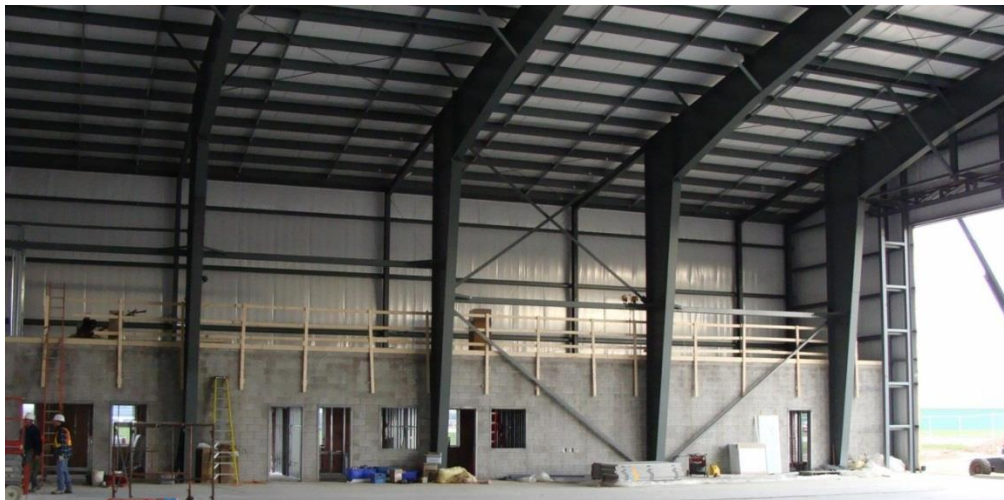
Interior main frames and 20'x104' mezzanine level
