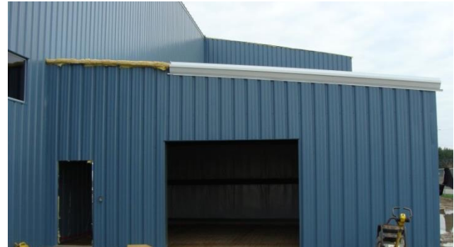
Ancillary building (30'x25') endwall elevation (roadside) with exterior cladding installation being completed
