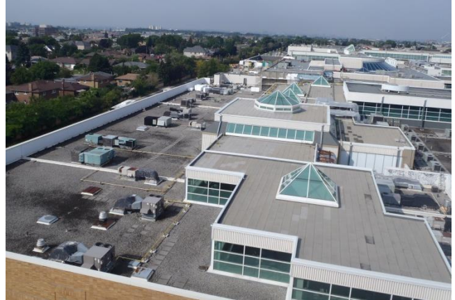
On-Going Rehabilitation of Roofing Systems Utilizing a Sustainable Long Term Lightweight Insulated Concrete System
