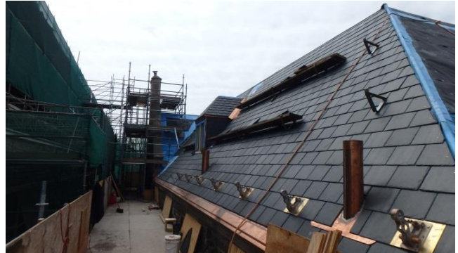
New Slate Roof and Copper Flashings at the Rectory
