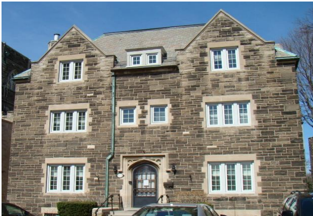
Rectory Building Prior to Stone Cleaning
