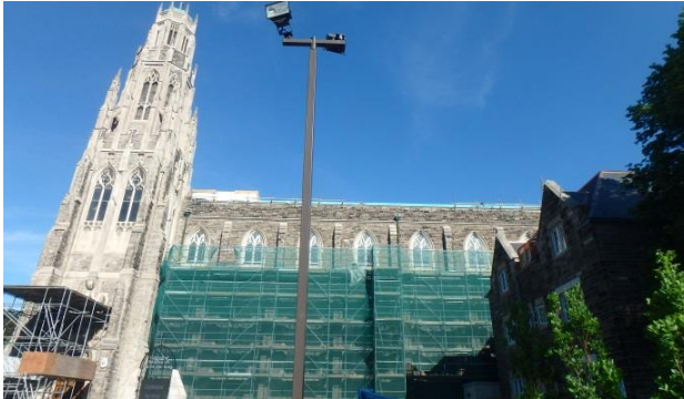
Scaffolding and Access Masonry Repairs of Cathedral
