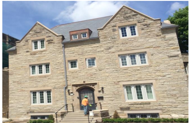
Rectory Building After Stone Cleaning to Remove Stains and Pollutants
